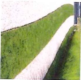
Planted ribbon natural concrete driveway
