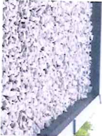
9mm grey stone chips on derbigum
