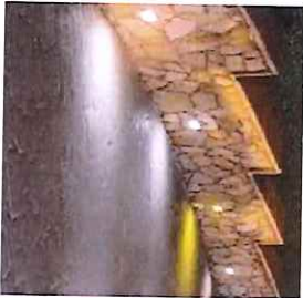
Low mounted wall light
